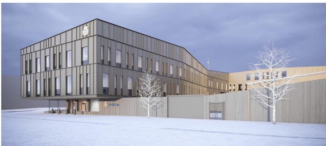
Illustration of the new police station that SBB is constructing for the Swedish police in Kiruna.
