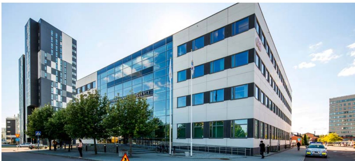
The Samuel 2 property in Västerås
